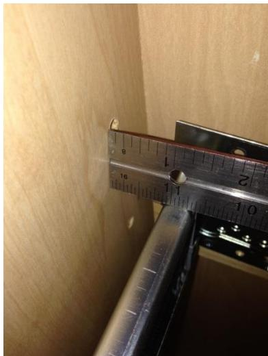
**TIP** While you are in the cabinet, measure the distance from the wall of the cabinet to the slide. The rear mounting socket is designed to float left to right. Sometimes the mounting socket is tight and you may need some force to move it. The slides should be equidistant from each side.
