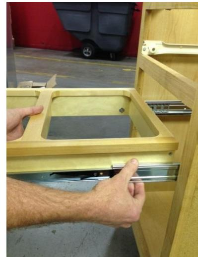
Step 6 Carefully push the top mount frame into the cabinet. There will be some resistance to re-set the soft close mechanism. Fully cycle the frame a few times to make sure it is working correctly.
