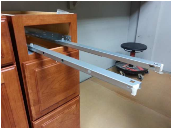
Step 3. Cabinet HW installed and extended
